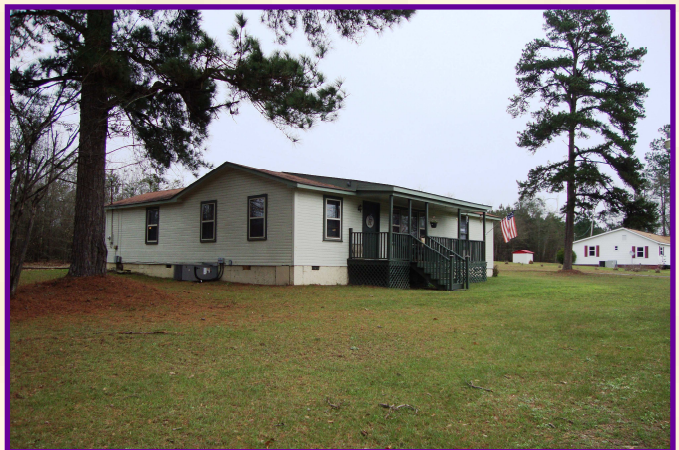
Additional view of home
